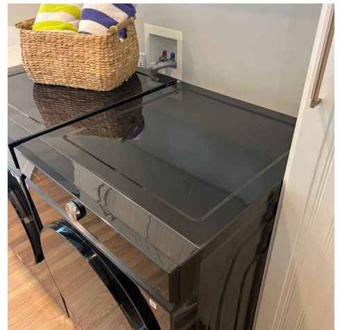
Dryer vent connected
