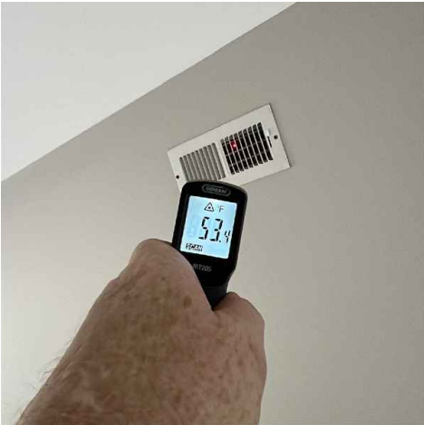
Second floor AC temp- House
