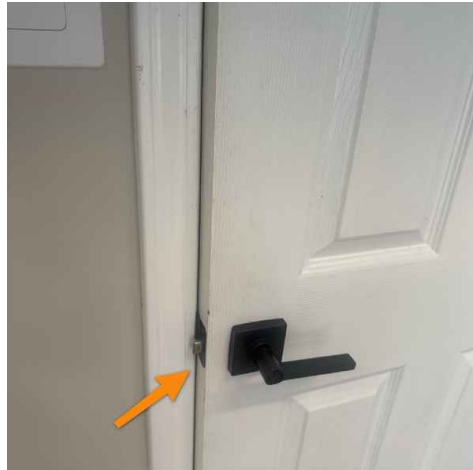
First floor powder room detached apartment
