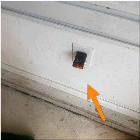
Attached garage right wall
