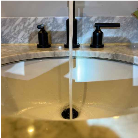
Sink disconnected from countertop
