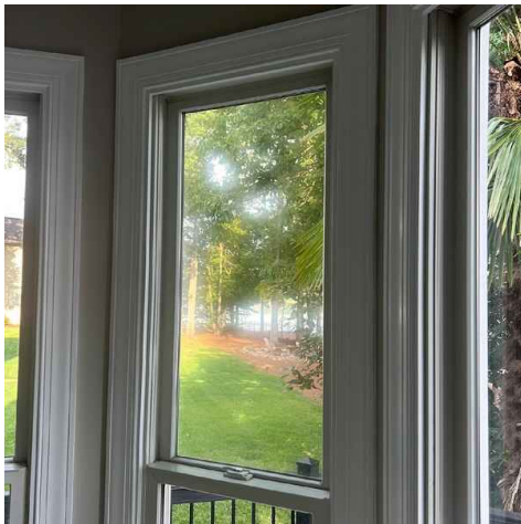
Master bedroom rear wall upper left
