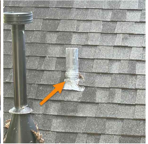
Outside bonus room attic
