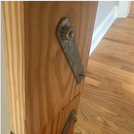
Left side attic stairs
