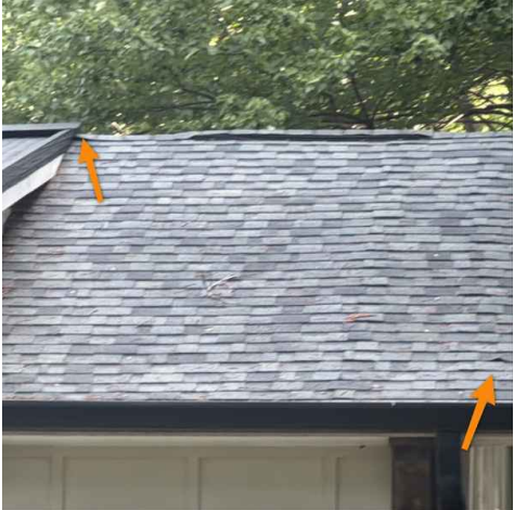
Apartment / garage roof
