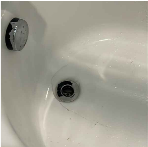
Tub drain stopper missing
