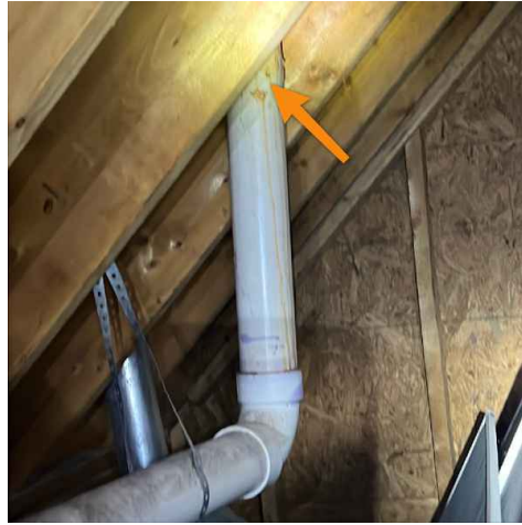
Inside bonus room attic
