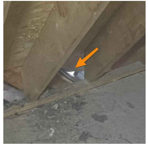
Right rear attic
