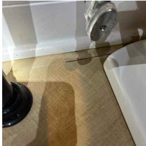
Behind master toilet
