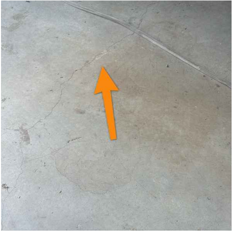
Garage floor left side
