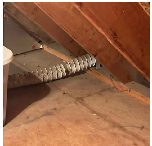
Left attic space second floor
