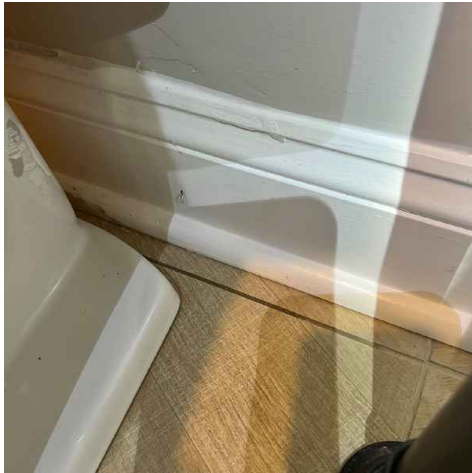
Behind master toilet
