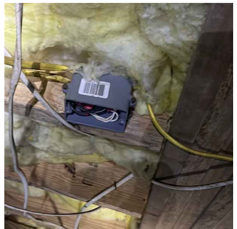
Left side crawlspace
