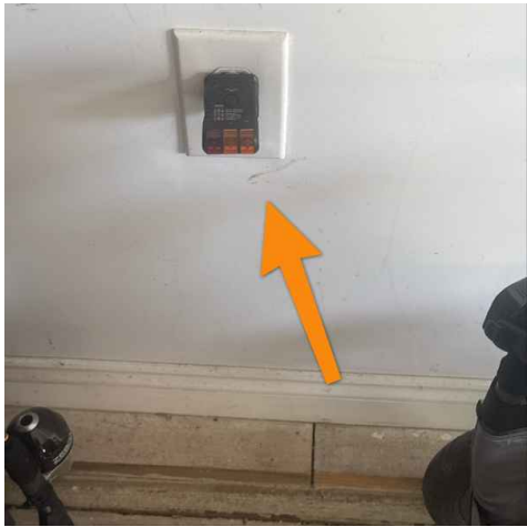
Attached garage right wall
