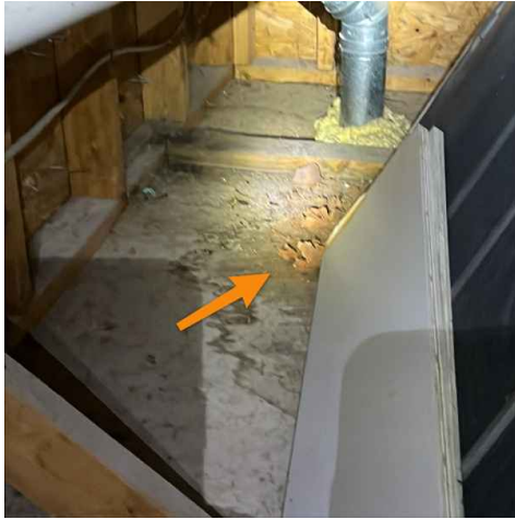
Inside bonus room attic
