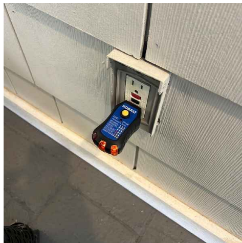
Rear back wall- Screen room GFCI
