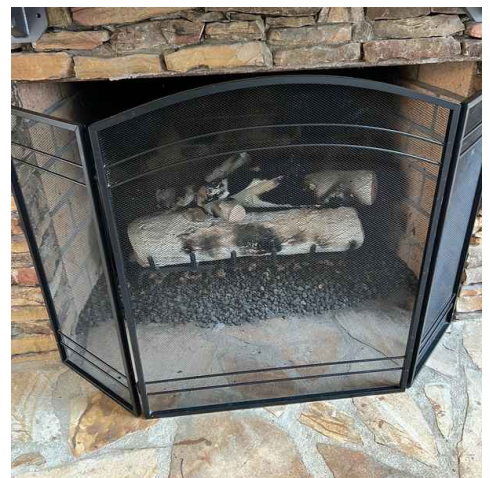
Living room gas fireplace
