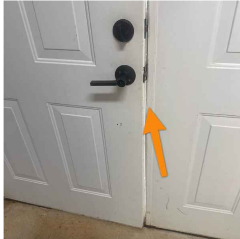
Apartment / garage rear door
